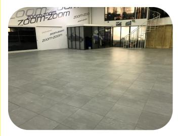
weberfloor 4310 fibre flow can receive foot traffic after just 2-4 hours and can be tiled after 12-24 hours, dependent on the ambient temperature following installation. The fibre reinforcement aids durability and allows it to be used in conjunction with under floor heating systems and floating floors. weberfloor 4310 fibre floor has excellent spreading and smoothing characteristics. It has low alkalinity and low emissions during drying and is casein-free.
